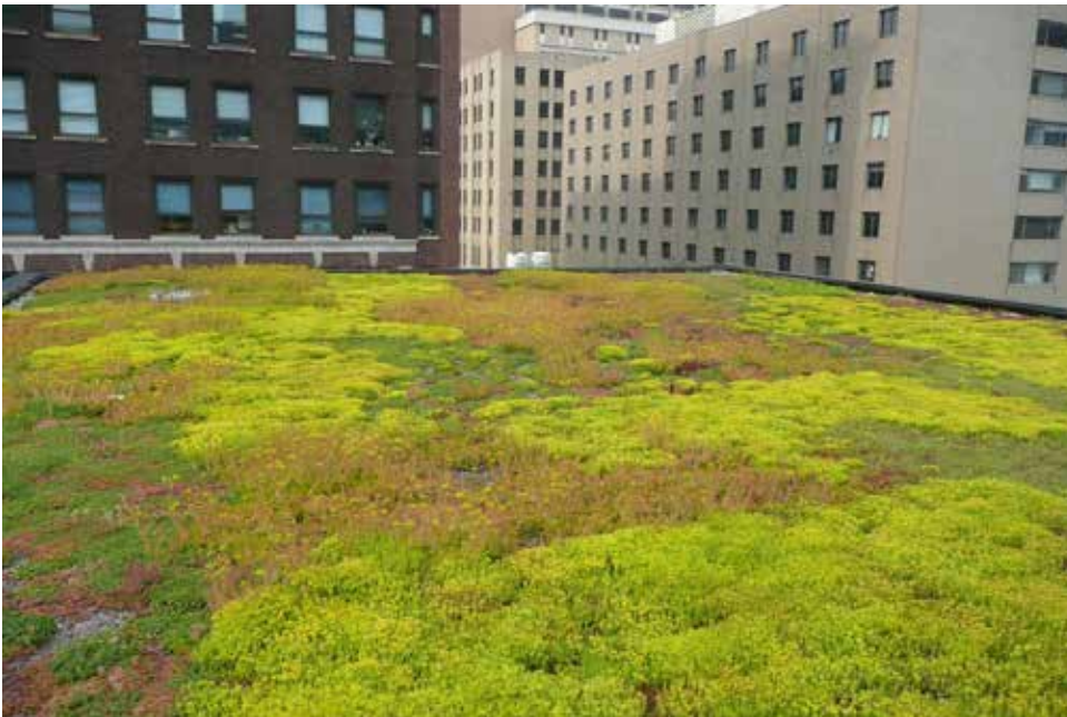
Figure 7.9: Green roof on an urban building.
